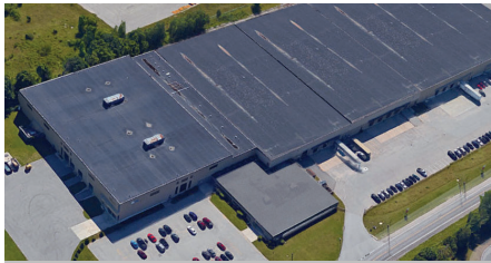
Barrie, ON (CAN) - High Performance Doors
